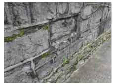
Fig.23 RB04 Stone decay and strap pointing
